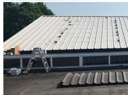
*A profile of the easy-to-install ClickFit EVO steel roof system (top photo). The bottom photo shows the custom-made rails that the installation specialist uses to snap and fix the solar panels in place.*
