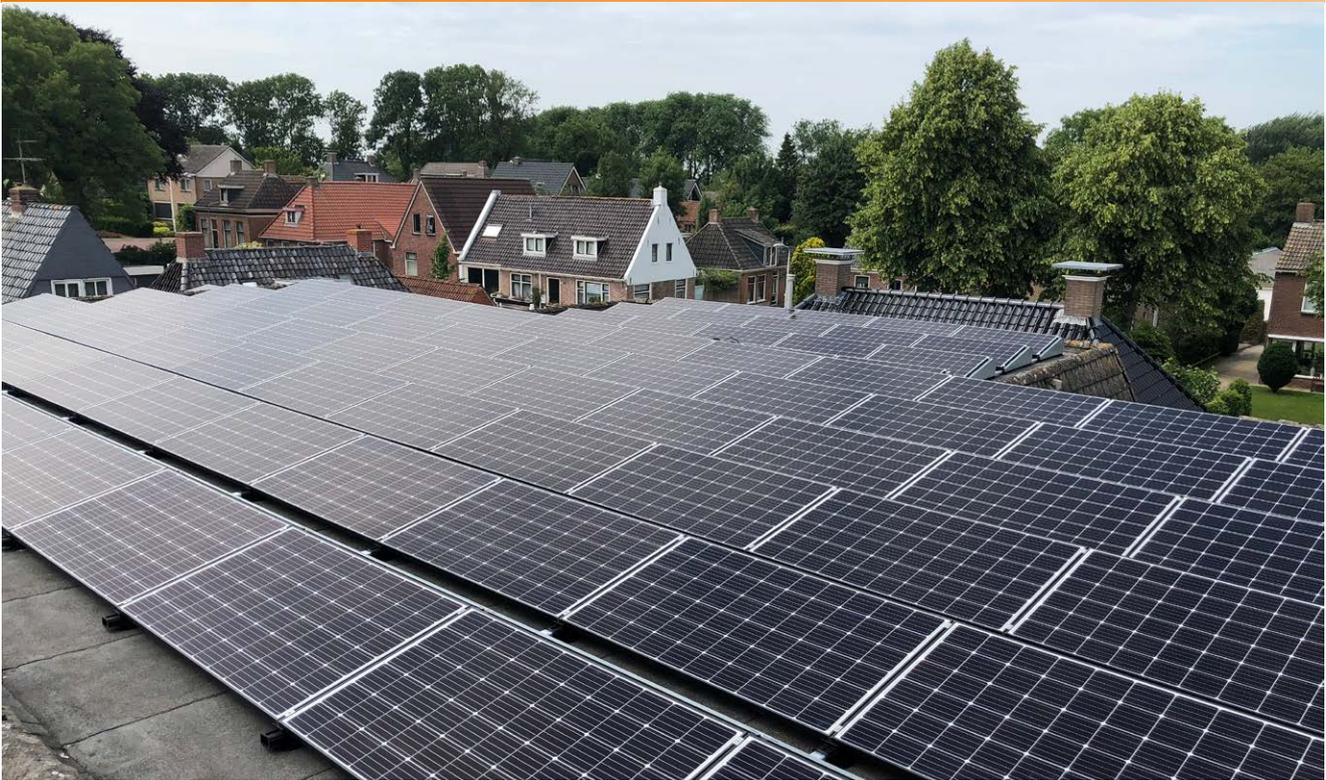
*A total of 400 solar panels have been mounted to two flat roofs, using the FlatFix mounting system.*
