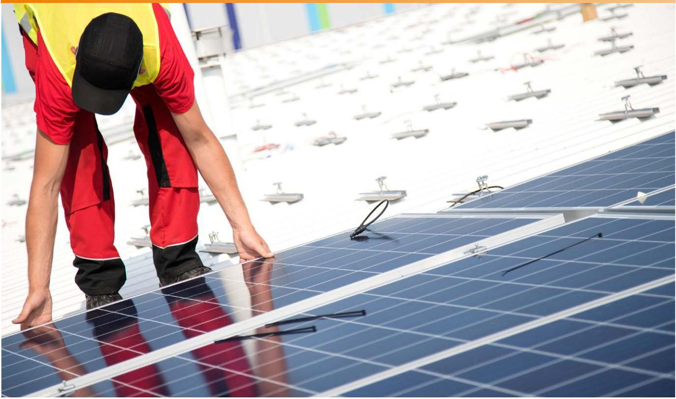
*NoCo2 technicians can easily snap the solar panels into the profiles of the ClickFit EVO system.*
