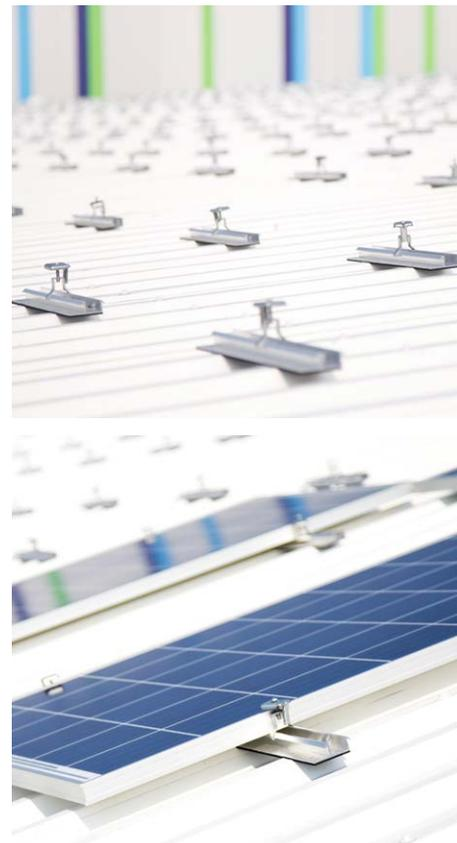
*Profiles of the ClickFit EVO mounting system on the steel roof in Hoogezand. Ultimately, 3,150 solar panels will be installed here.*
