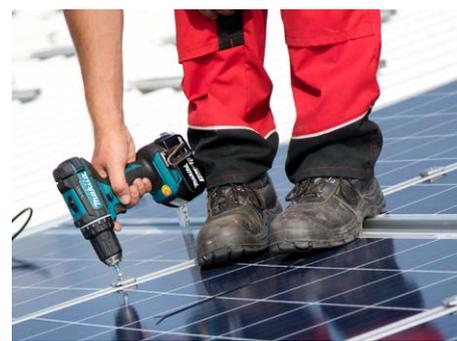
*The panels are attached to the rails with a special, universal modular clamp.*
